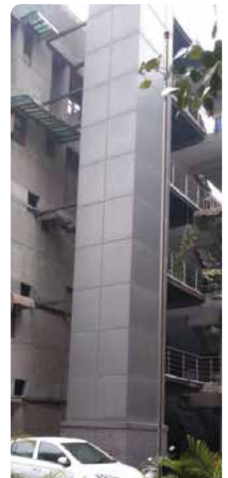
Actual Site Image of Structure lift with ACP Sheet Installed in Narmada Apartments Delhi
